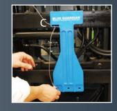
5. Pull free end of the leash down through the hole at the top of the Blue Guardian (C) to bottom of the Blue Guardian and insert between the bumper and the frame.
