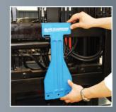
and slide a standard sized pen (12 mm) under the Blue Guardian frame. If the pen does not pass under the Blue Guardian, there is not adequate floor clearance and the Blue Guardian should be
